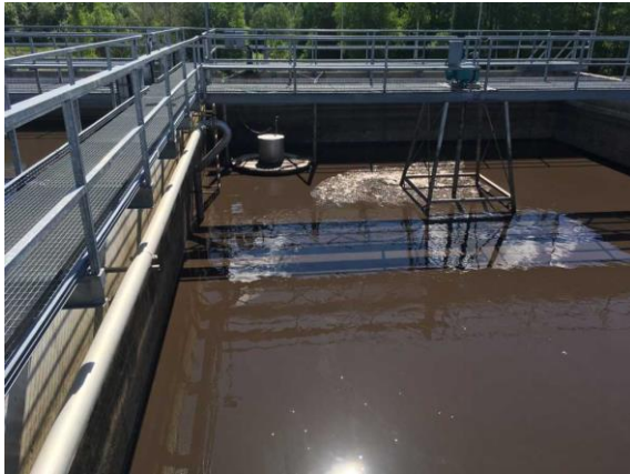
Figure 4: SBR with mixer and decanter
